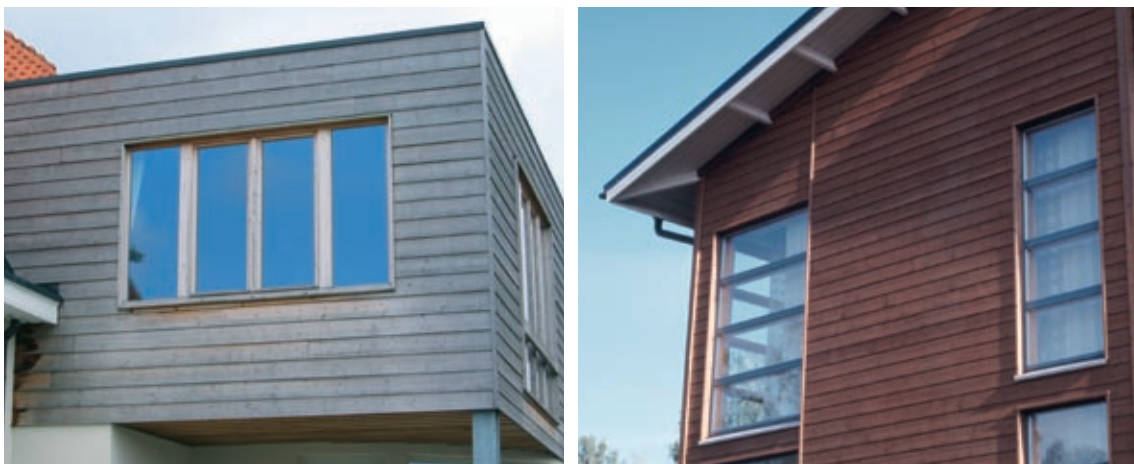
Two examples of ThermoWood cladding after three years weather exposure with and without surface coatings.
